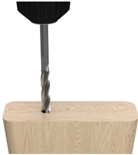
1. Drill two holes straight into the leg (Recommended hole size \text{Ø}7 \times 70 \text{ mm} )
